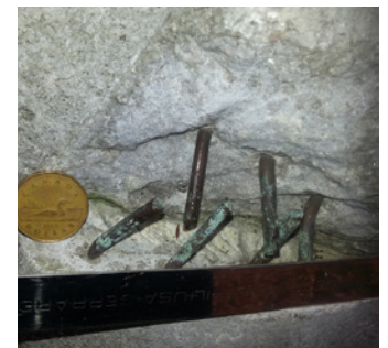
A metal band around the collection of four "provincial panels" has damaged the Arctic panel by sculptor Emanuel Hahn. The limestone around the figure's torso has worn away exposing metal underpinnings.
