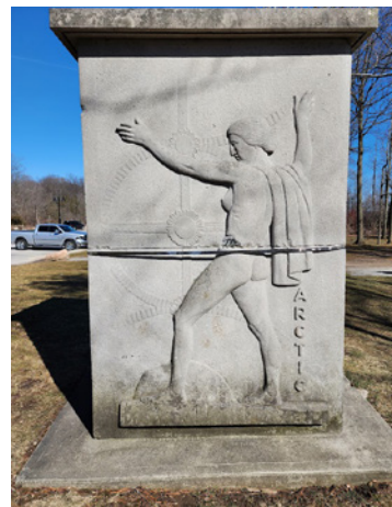
A metal band around the collection of four "provincial panels" has damaged the Arctic panel by sculptor Emanuel Hahn. The limestone around the figure's torso has worn away exposing metal underpinnings.
