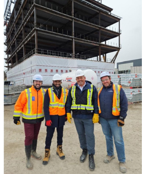
I had the opportunity to visit the construction site for the medical school building at UTSC.
